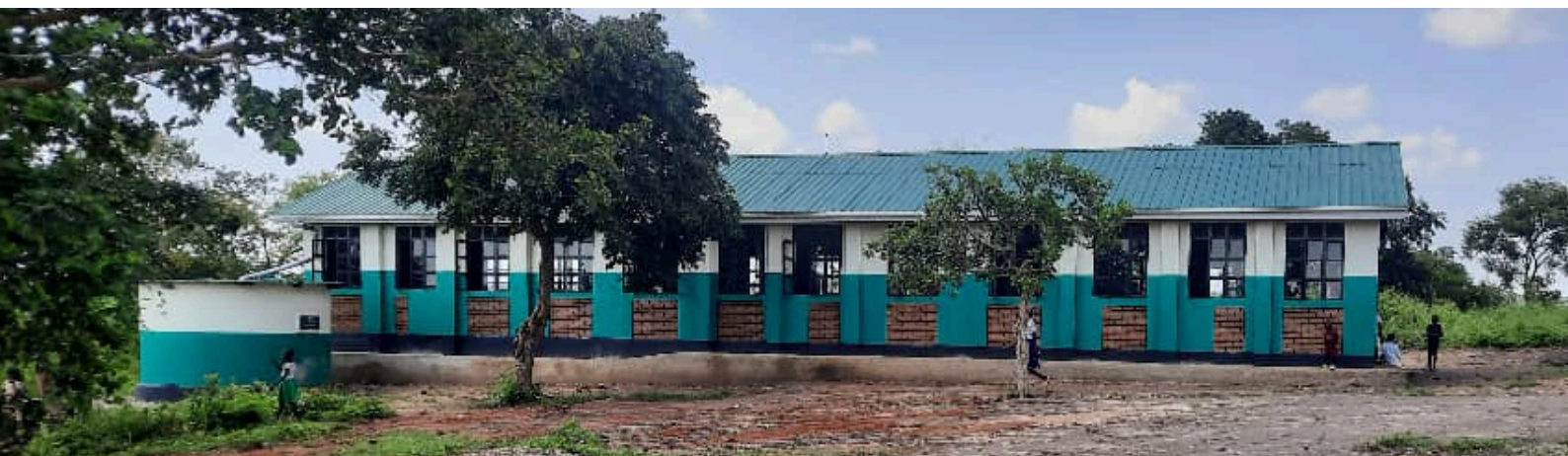
New infrastructure at Morimo Primary School, Koboko District
